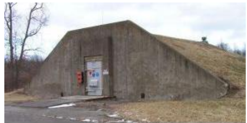
One of 99 bunkers built at Plum Brook Station by the Army during WWII, currently used and operated by the Glenn Research Center (GRC). Source: IG Report.
