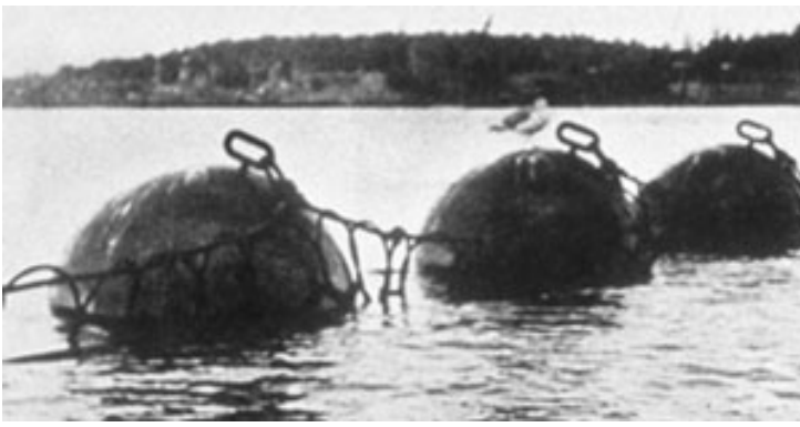
Figure 1. Submarine nets consisted of chain gates weighted by concrete at the bottom and supported by buoys.
