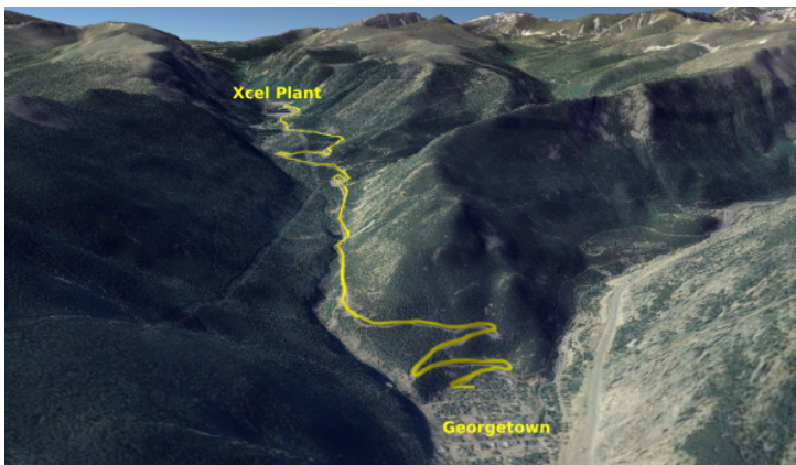
Figure 3. Georgetown, CO, is a 15-minute drive away, not including the off-road, up-hill path to the upper reservoir. Source: CSB
