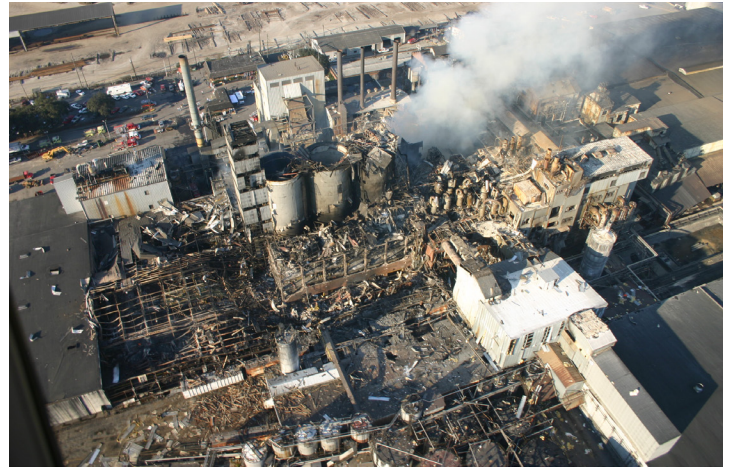
Figure 1: Imperial Sugar Company's refinery in Port Wentworth, GA, suffered catastrophic damage when combustible sugar dust exploded.
