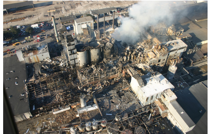
Figure 1: Imperial Sugar Company's refinery in Port Wentworth, GA, suffered catastrophic damage when combustible sugar dust exploded.
