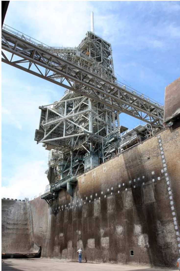
An inspector examines the repaired section of the flame trench wall.
