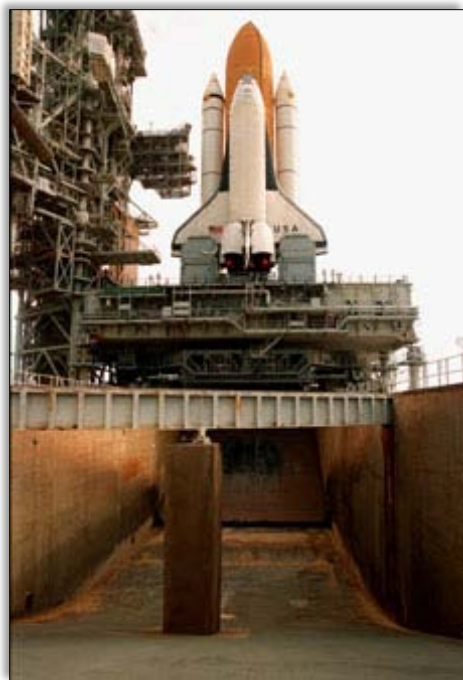
The flame trench of Pad 39A
