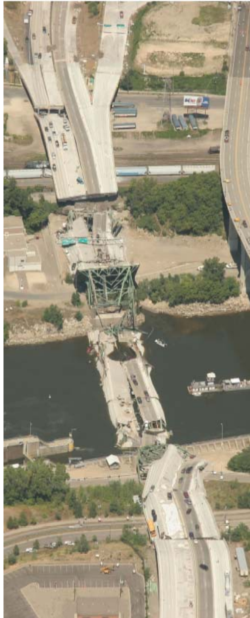
Figure 4: I-35W Bridge on August 2, 2007, the day after the collapse
