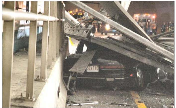
Figure 1: The passenger seat was completely crushed by the fallen concrete panels.
