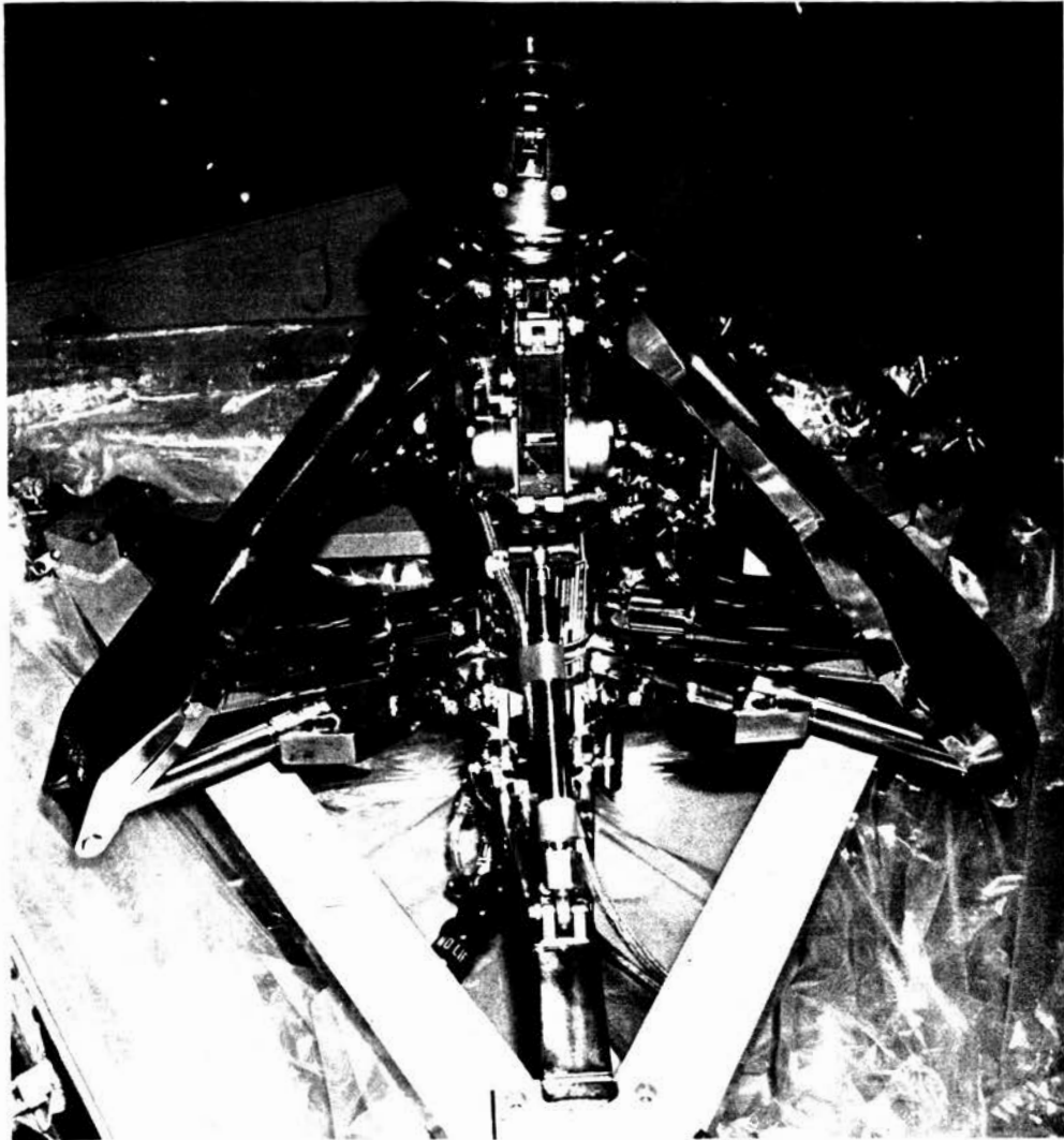
Figure 1.- Apollo 14 probe assembly.
