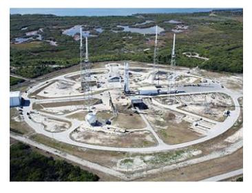
Falcon 9 launches from Cape Canaveral use Space Launch Coi 40. Originally built in the 1960s for the Titan IIIC rocket, the lau of SpaceX CRS-2 is the sixtieth launch from the pad. Fifty five rockets; Twenty six IIICs, eight 34Ds, four Commercial Titan III seventeen Titan IVs; flew from the complex.
