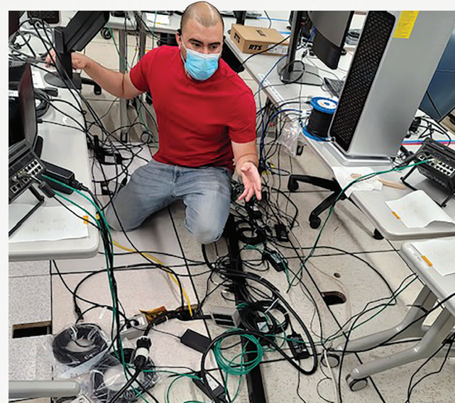
The Jet Propulsion Laboratory: Luis Gaitan organized months of sloppy power and signal cabling for the NASA-ISRO Synthetic Aperture Radar. He safely routed the cabling that wasn't removed to the SAF-122 control room.
